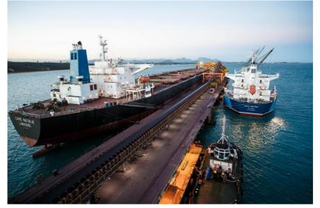
It is also connected to the tugboats' pier (located along the East side and capable to accommodate two 28m LOA tugs alongside in line which, in turn, are able to accommodate another two tugs of the same size.
