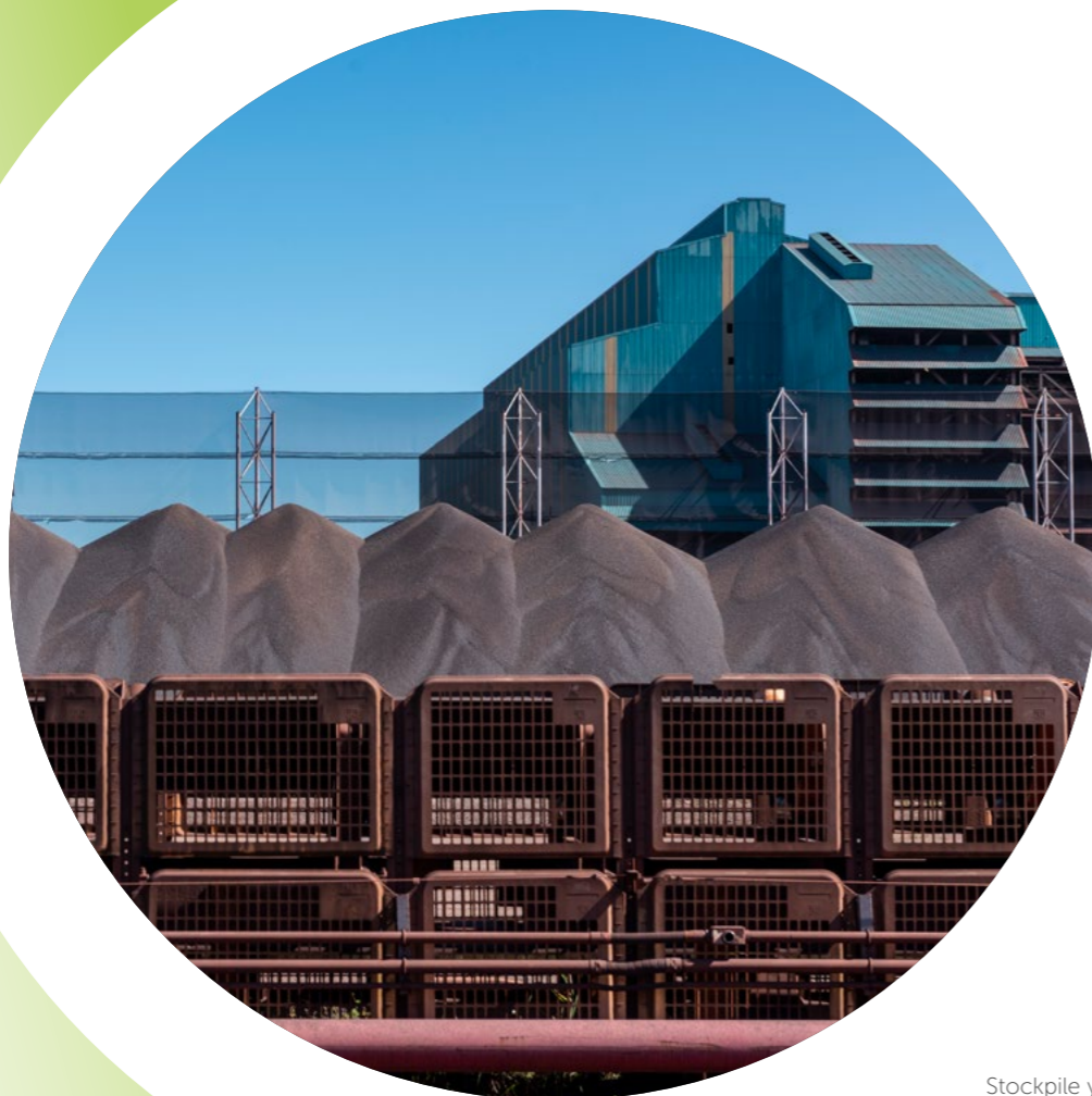
Stockpile yard and plants, Ubu Complex (ES)
